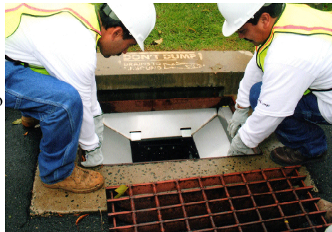
DPW workers installing filter
